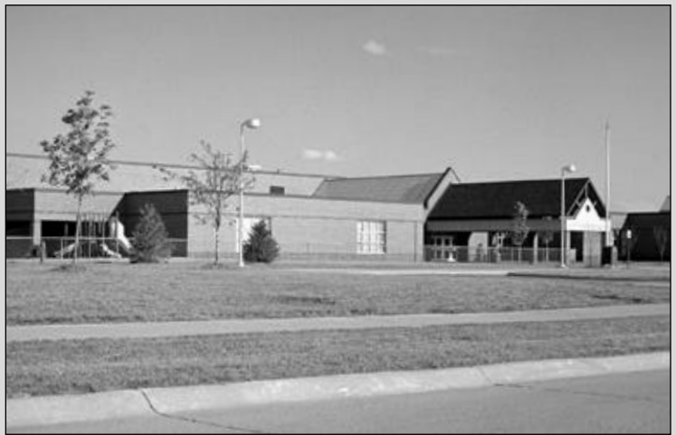
Cavett Elementary School in Lincoln, Nebraska, is one of several Lincoln schools that saves money and energy with GHP systems.
